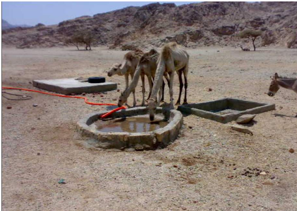
The Solar Pumping System for Bedouins Communities
