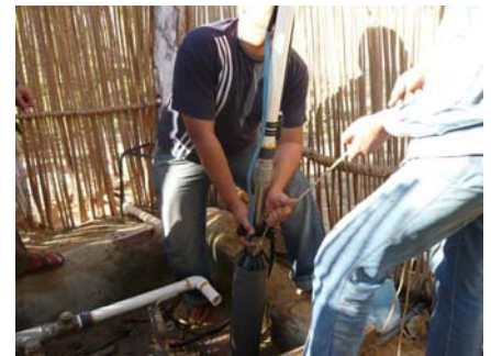
Pump Well Installation
