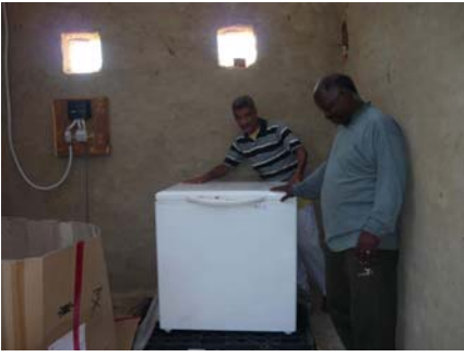
ECO Lodge Staff Use the Solar DC Refrigerator
