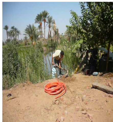
Pump Cable Connection Process
