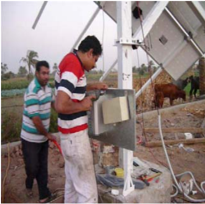
Electrical Panel Installation
