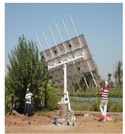
Final PV Install
