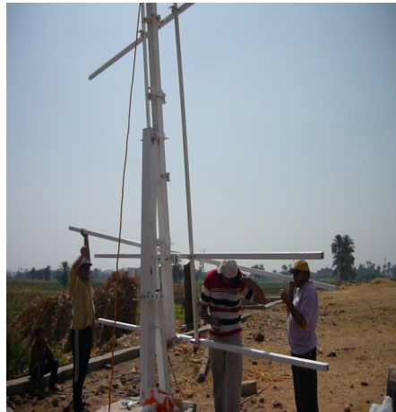
Track Assembly Process
