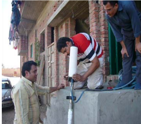
Pump Preparation Process
