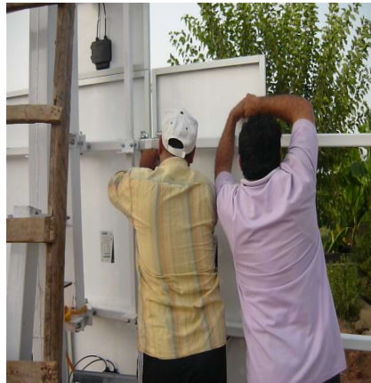
PV Install Process
