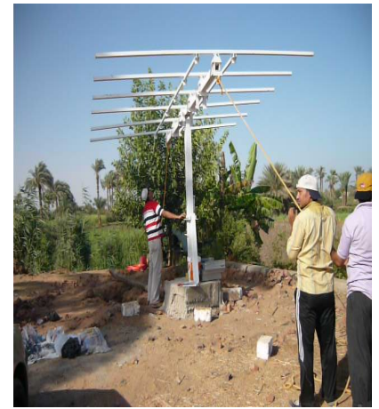
Final Track Assembly
